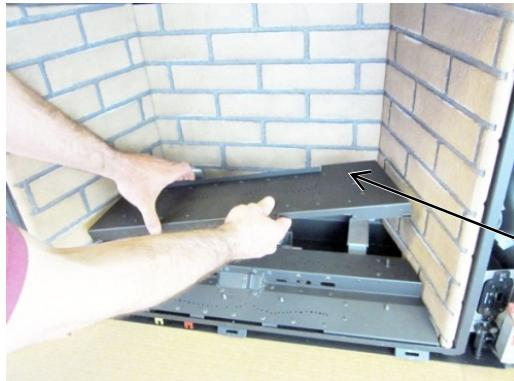
NOTE: Remove the attachment screw first.
